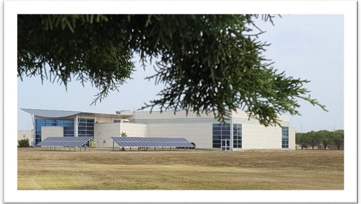
Solar array on the Kansas State University Polytechnic campus
