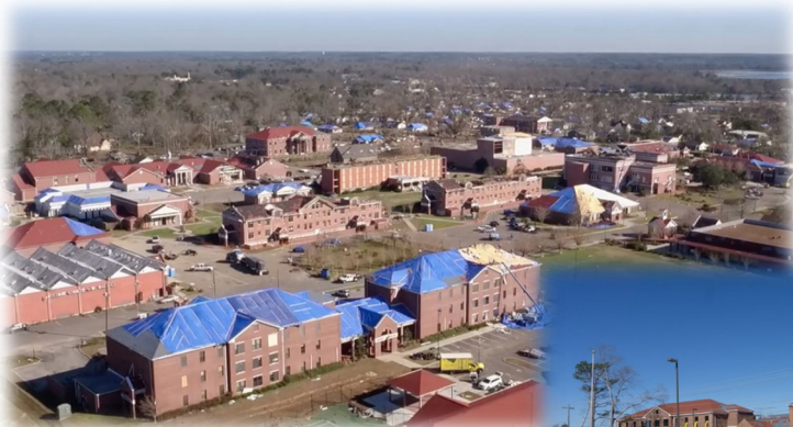
William Carey University suffers severe damage to 40 campus buildings.
