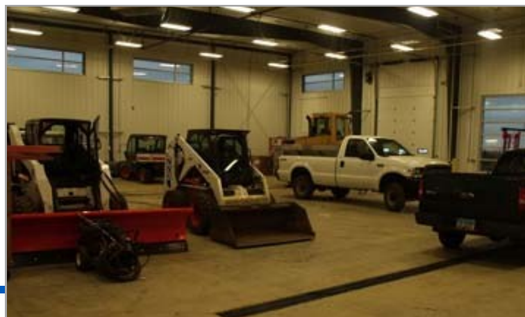
BSC provided the photos of the nearly completed facility, shown here.
